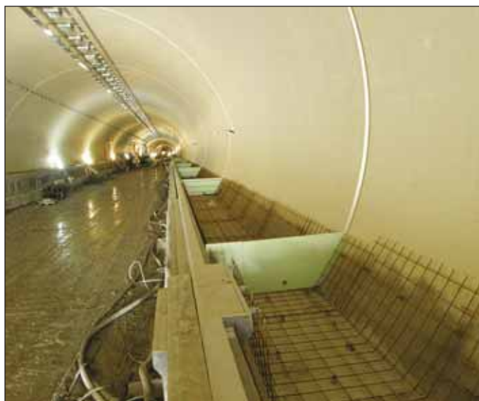
Obr. 7 Betonáž chodníkov tunela Fig. 7 Casting of tunnel walkways
