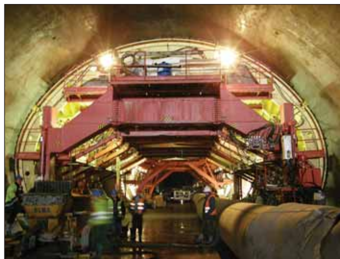
Obr. 6 Betonáž sekundárneho ostenia tunela Fig. 6 Casting of the secondary tunnel lining
